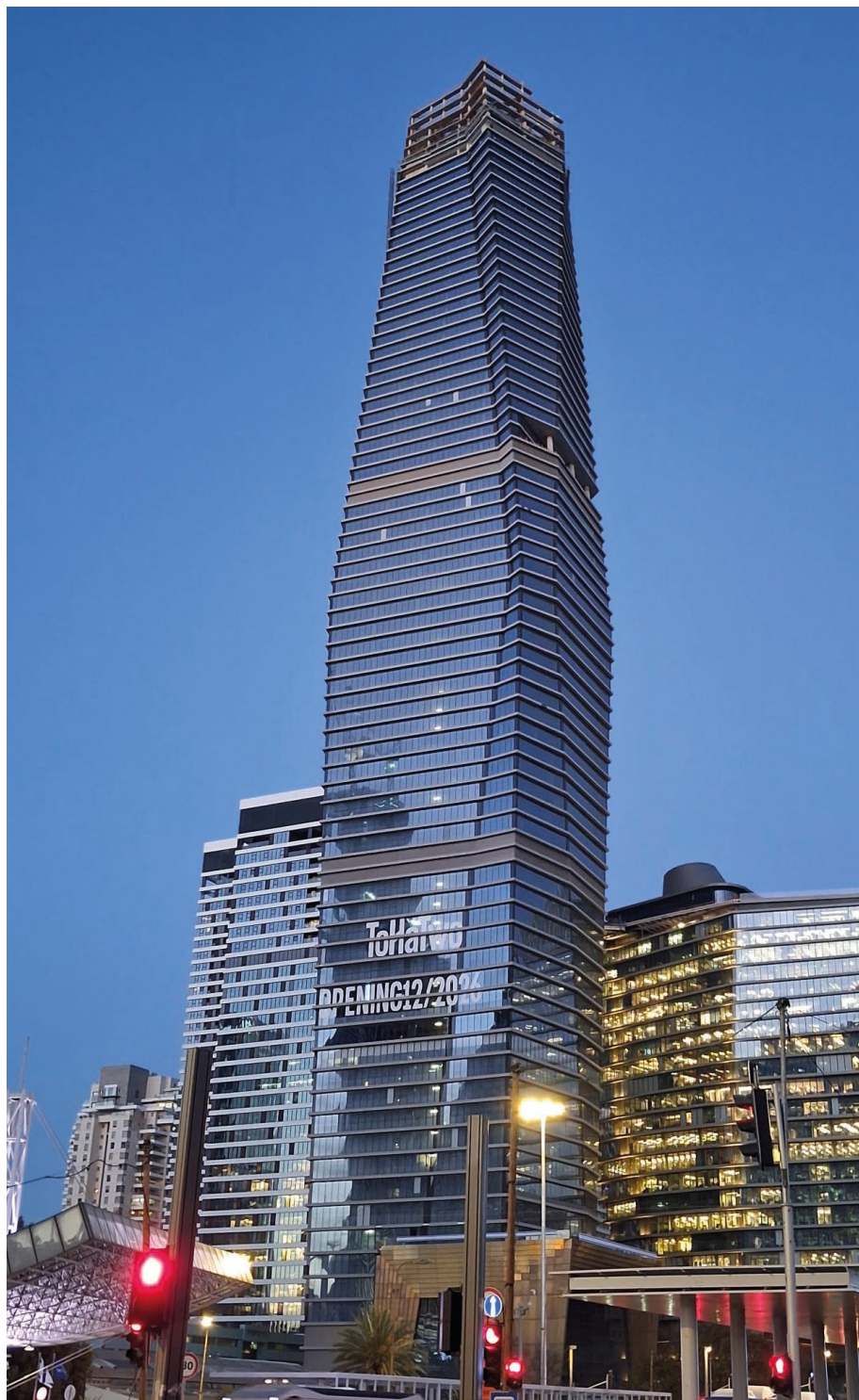
ToHa 2, rising to about 298 metres, the third tallest in Israel, anchored by Google's record lease at the city's eastern gateway. Source: Wikipedia/Mister Gvartsian under Creative Commons CC0 1.0
